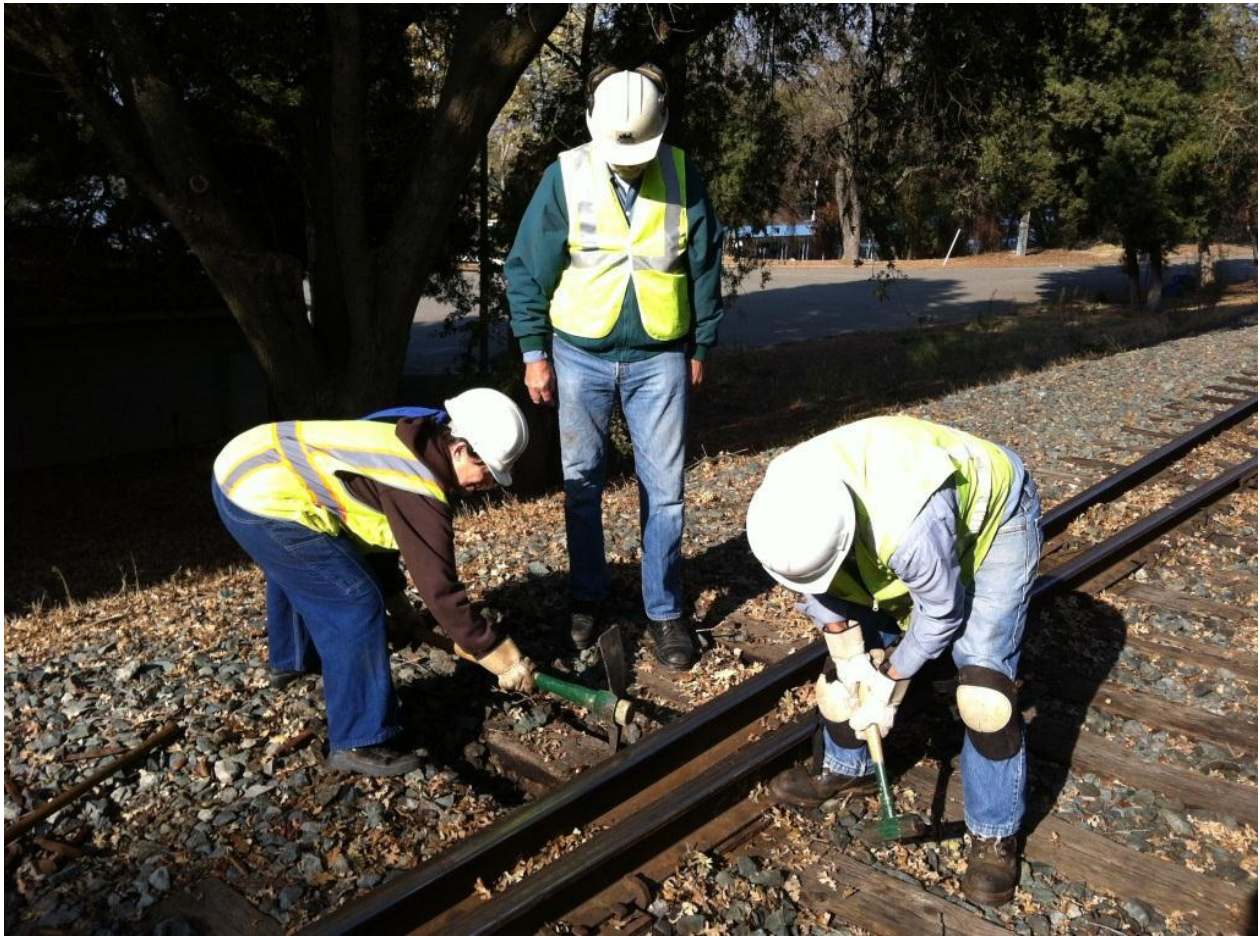
Alan supervises Pam and Mike T. pounding out the tie plate on the switch tie being replaced
